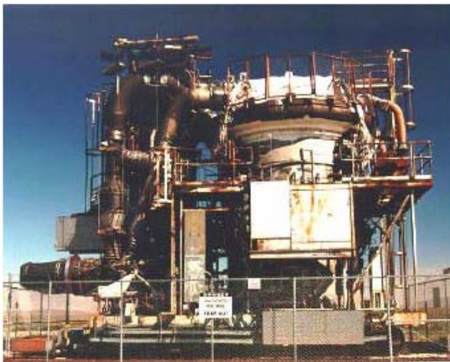
Figure 1-2 Core Test Facility
