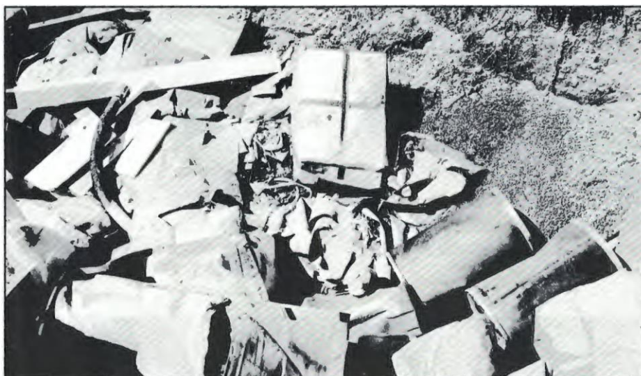
Notes for above RWMC photo: Waste in a disposal trench, 1962. Many of the waste containers have disintegrated, leaving loose waste scattered around the trench. (DOE-ID Photo 62-2134)
