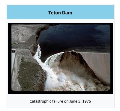
"The **Teton Dam** was an <u>earthen dam</u> on the <u>Teton River</u> in <u>Idaho</u>, United States. It was built by the <u>Bureau of Reclamation</u>, one of eight <u>federal agencies</u> authorized to construct dams.<sup>[3]</sup> Located in the <u>eastern part</u> of the state, between <u>Fremont</u> and <u>Madison</u> counties, it suffered a catastrophic failure on June 5, 1976, as it was filling for the first time.
