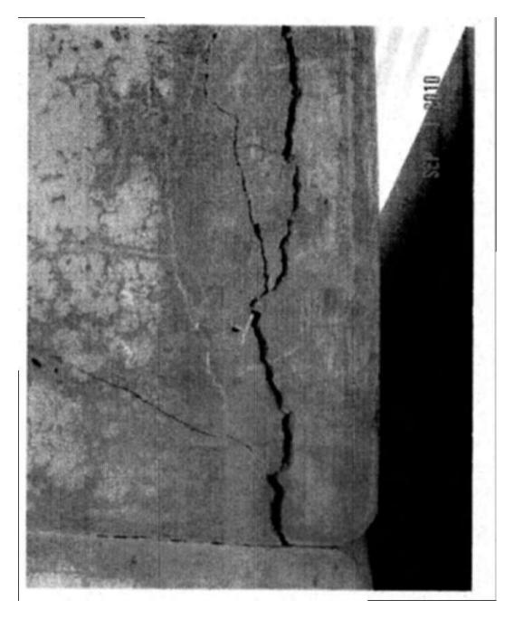
This picture is of unexpected cracking of concrete, prior to repair, from the 2012 NRC inspection of the Three Mile Island independent spent nuclear fuel storage installation at the Idaho National Laboratory.
